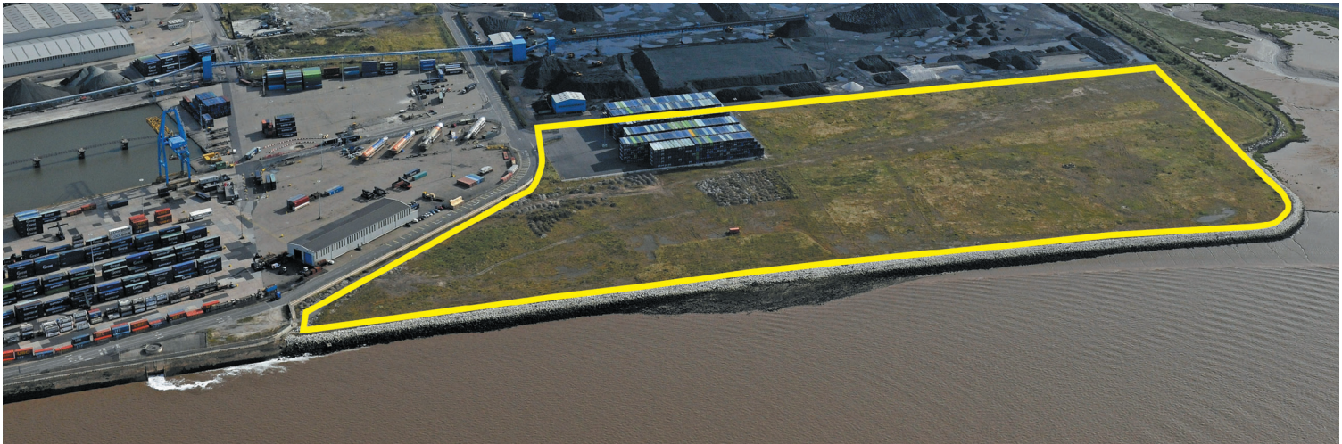
PROPOSED SITE FOR THE BIOMASS POWER STATION NEAR QUEEN ELIZABETH DOCK, PORT OF HULL
